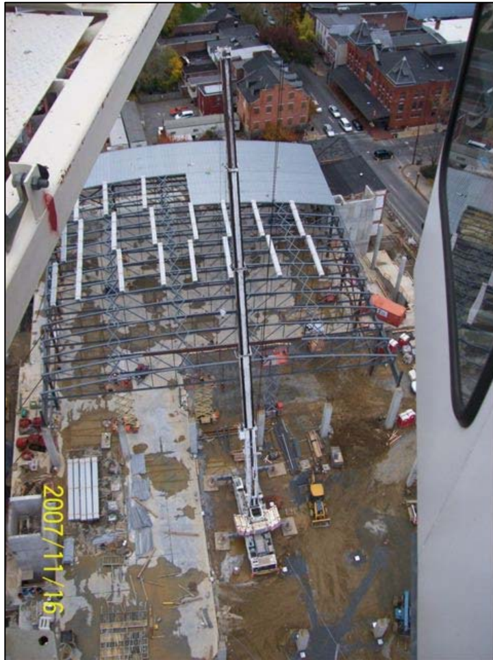
Figure 18 Steel Erection
